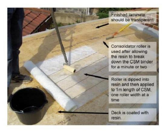
Unroll the mat on to the resin coated board. In strips of 7" (1 roller width) wet out the mat by dropping 1 roller full in the middle of each 7" run, push the roller away to the end of the 1 metre run, then pull back over the full 1 metre. This will ensure even coverage.
