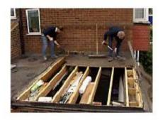
After removing the old decking, check that all roofing joists are sound and free from rot. Replace these as required. If possible, build a fall into the substrate so that the roof can drain completely and remain free from standing water.
