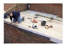
PU adhesive is applied with a skeleton gun to the batten around the perimeter of the roof. A 30mm bead at 300mm centres is sufficient to hold the trims in
