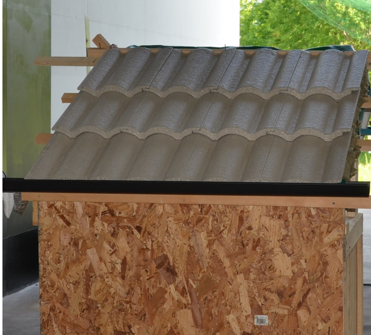
Figure 4. Concrete Tile Roofing Assembly (profiled tile) Exposed to Wind-Driven Firebrand Showers. The dimensions of each tile were 420 mm long by 320 mm wide. The Height, from the Wind Tunnel Floor to the Base of the Gutter of Roof Deck was 1250 mm.
