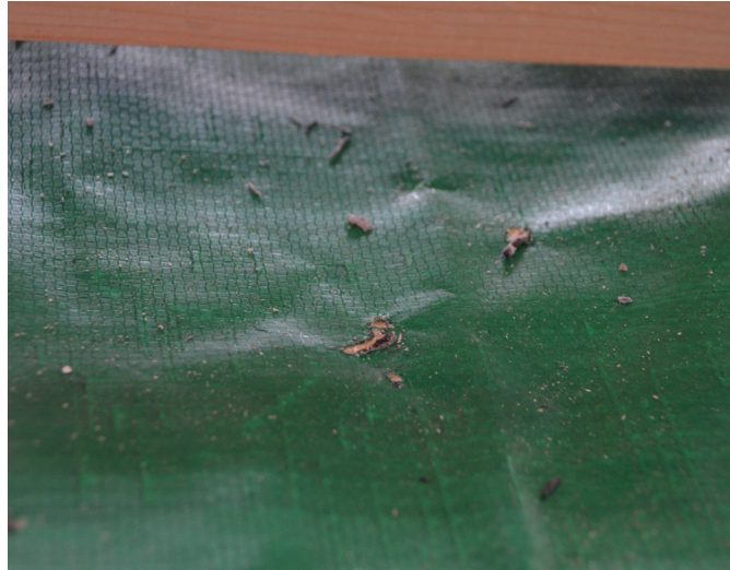
Figure 9. Images of Sarking Placed Under Concrete Tiles (profiled tile) Taken Immediately after the Experiment was Completed. The Tiles have been Removed.
