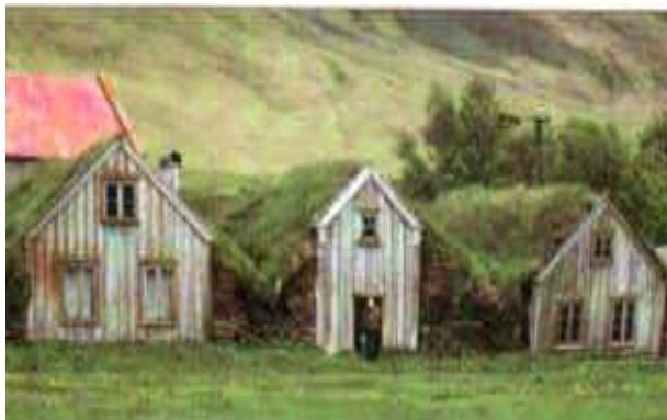
Figure1: Turf Roof (Magnusson 1987)
