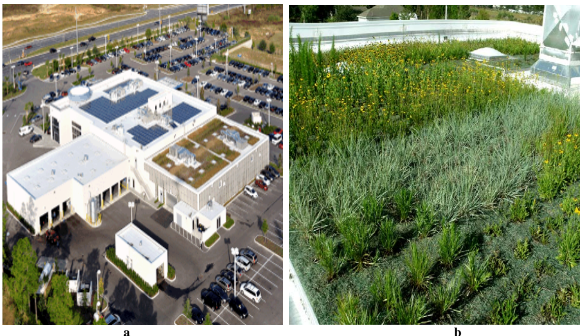
Figure 9: a showing top green roof and PV panels, b showing sedum and perennial plants ( www.greenroofs.com )
