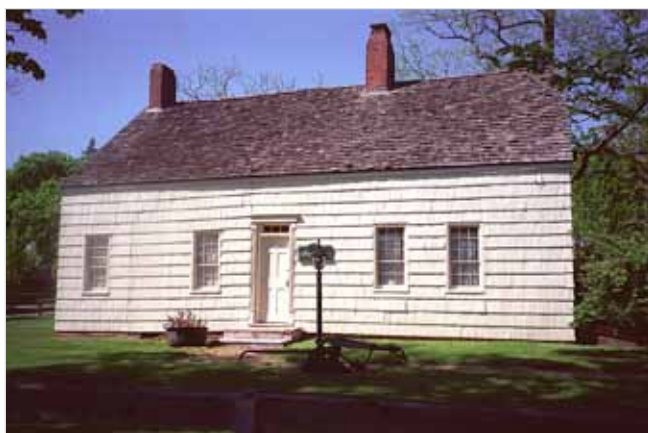
Figure 2. Example of shingle roof after decades of service.
