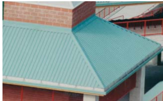
Metal roof - Jerry Uht Stadium, Erie, PA
