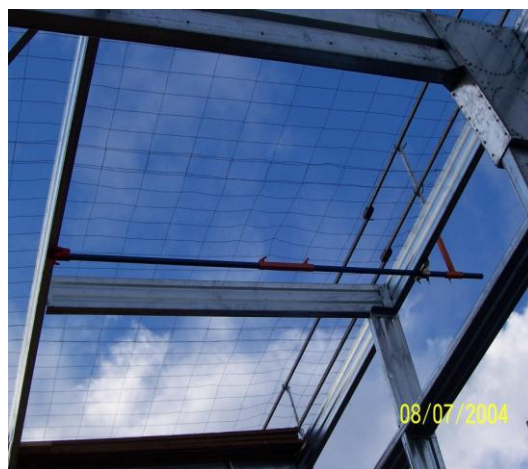
Figure 15: An example of safety mesh installed prior to roof construction.
