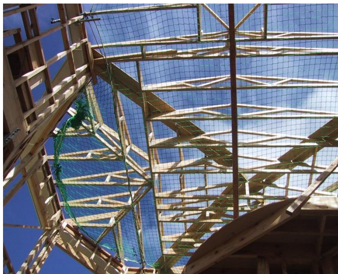
Figure 6: Safety nets set up under a roofing construction to catch falling workers, debris, or tools.
