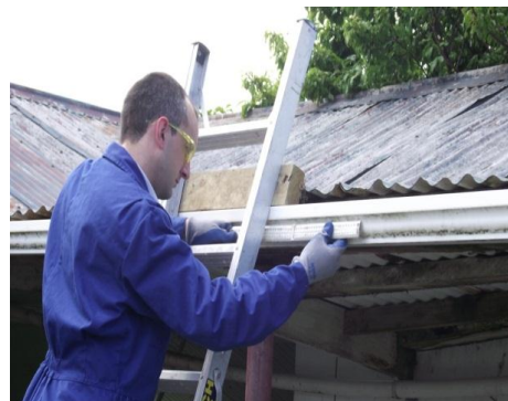
Figure 1: A worker maintains three points of contact while working from a ladder.
