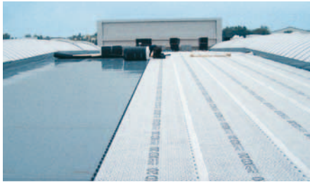
1. The roof membrane is covered with the protection, drainage and water storage element Fixodrain® XD 20 .
