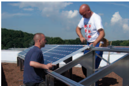
5. The solar panels are installed.
