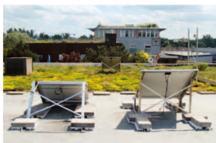
The difference in temperature of various roof build-ups was measured using a test installation on a ZinCo roof.
