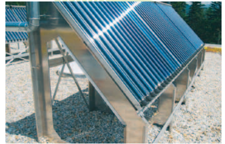
Base frames with a different angle are often used for solar thermal systems.
