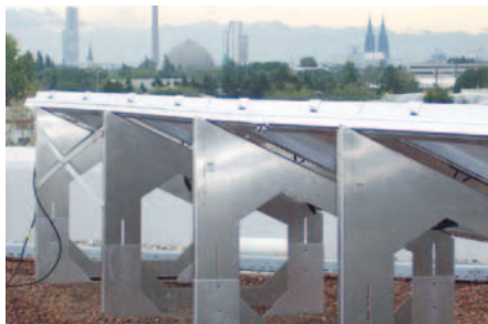
Height-adjustable Solar Base frame for levelling out the roof pitch (e.g. with thermal insulation incline).
