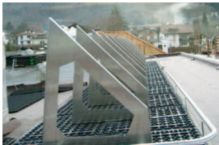
Frame 45° for solar thermal panels on a roof area with a 5° slope.
