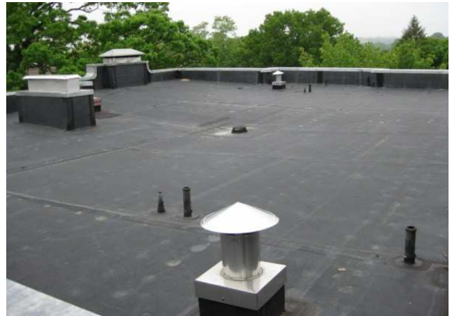
107-Single Ply Membrane WITH OR WITHOUT presence of gutters
