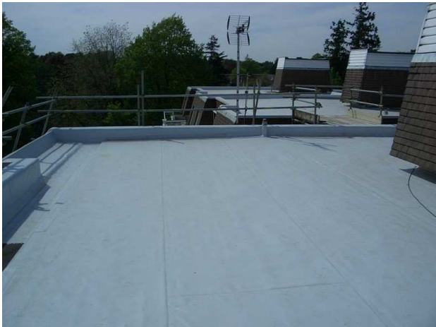
107-Single Ply Membrane WITH OR WITHOUT presence of gutters
