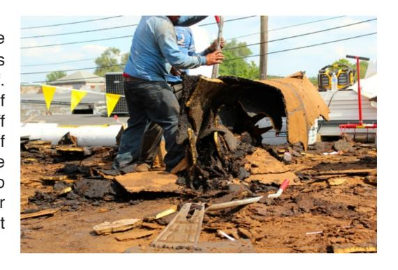
Don't be tempted to lay over top of or recover a saturated flat roof, it will cause you much trouble in the future. The trapped moisture will quickly rot out wood decking or rust out metal decks, the new roof won't last as long as it should and the next time your up for a tear off you'll be handling even more debris and layers of saturated flat roofing material.
