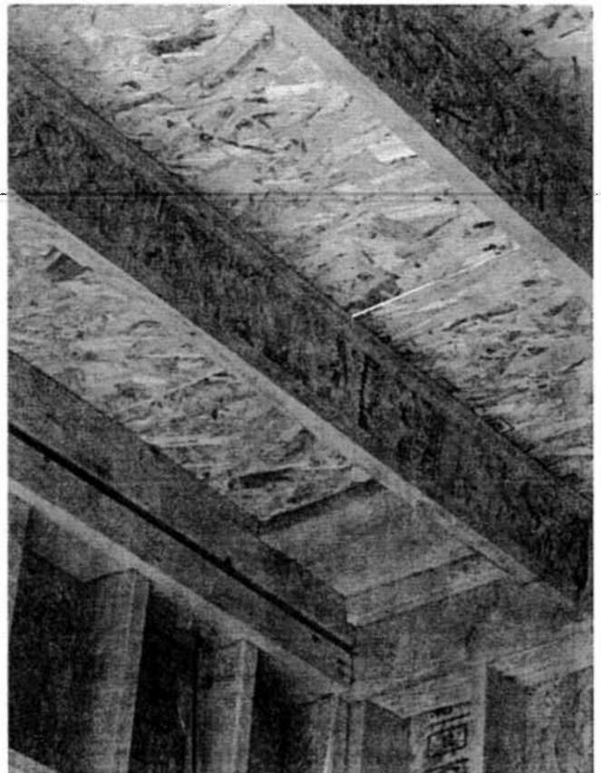
Fig. 22-39. Ceiling framing often supports a second floor.
