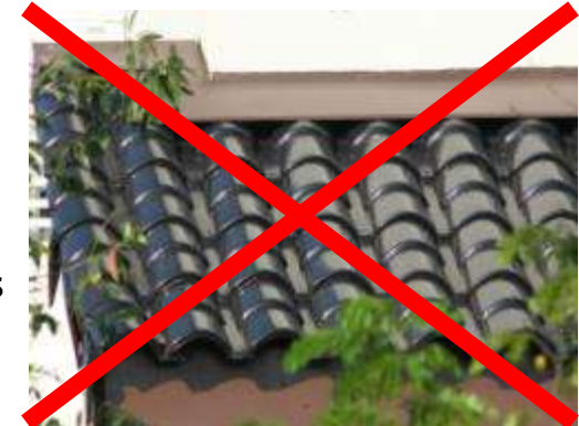
ZINC FLASHING AT ABUTMENT
