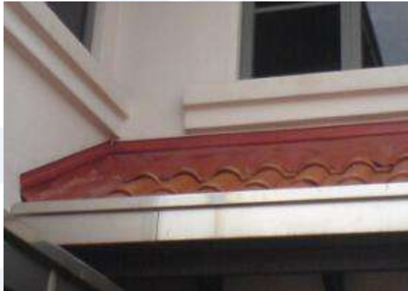
DRY FLASH AT ABUTMENT & PARTY WALL
