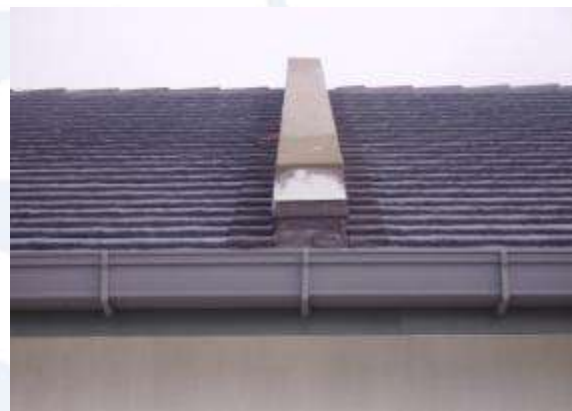
DRY FLASH AT ABUTMENT & PARTY WALL
