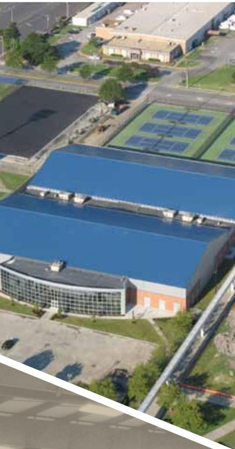
**BattenLok® HS** panels are 12" or 16" wide flat profile standing seam panels. Designed for reroofing existing buildings or roofing new ones of any type, the panels have 2" high ribs and are machine joined at the edges with a mechanically locking seamer. Lengths up to 45' are available and, longer panels may be ordered.
