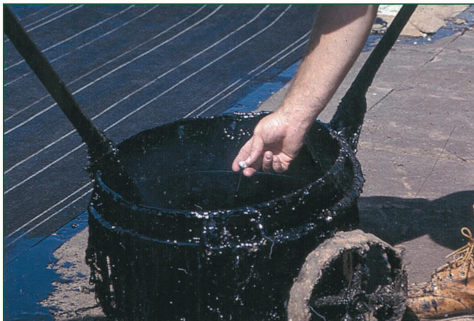
Photo 2: Asphalt temperatures need to be checked at the point of application.
