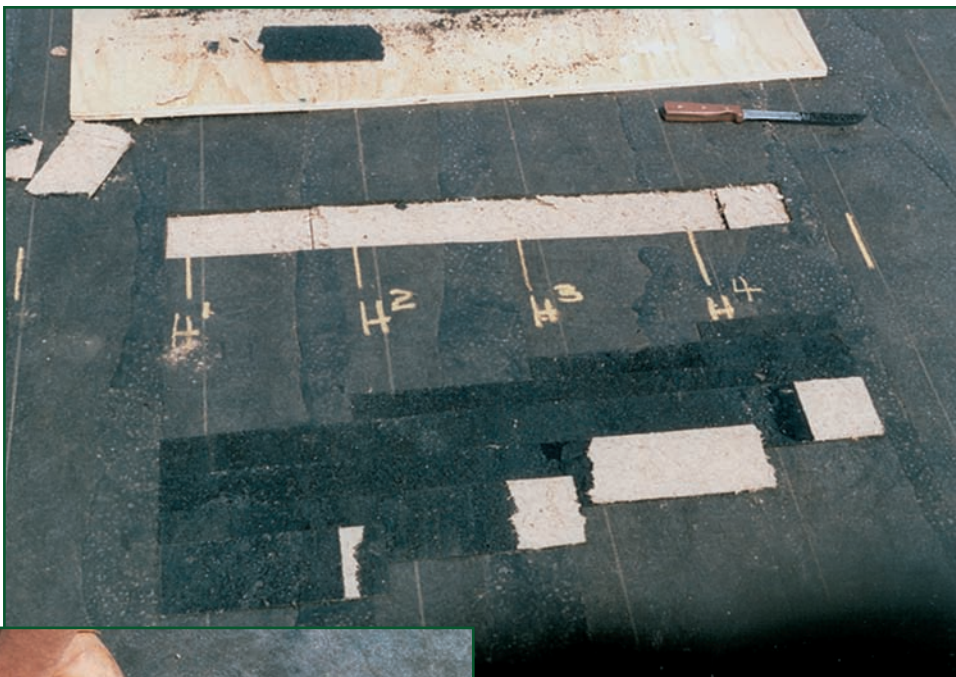
Photo 9: The relationship of individual felt plies to the sample area and measured headlap.
