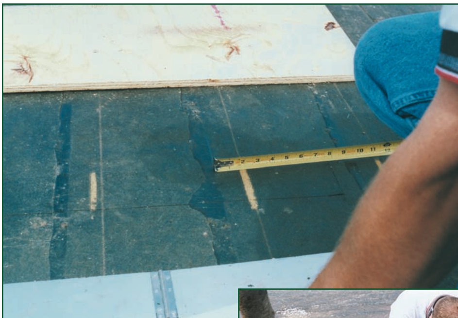
Photo 4: Measuring felt ply headlap in pre-determined sample area.
